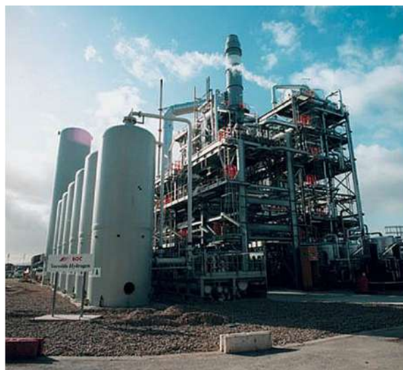
Figure 8.8 - Wood SMR Hydrogen Plant, North Tees
