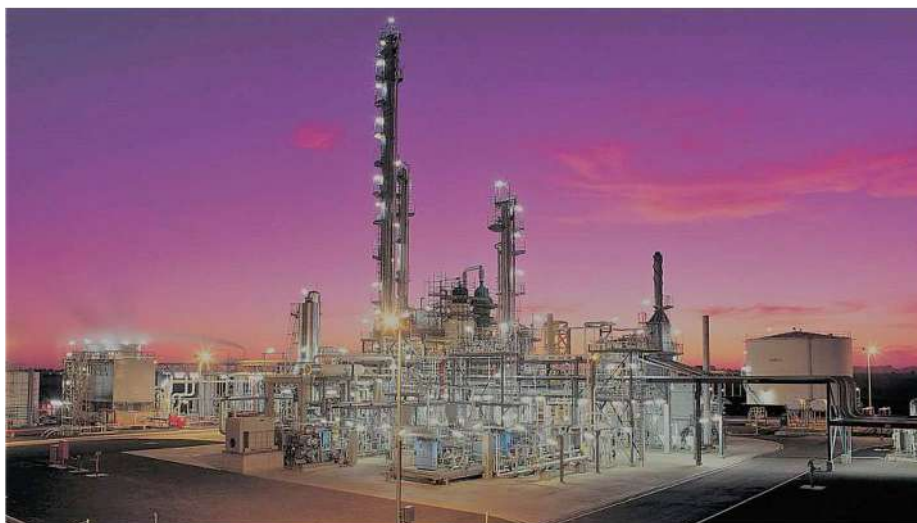
Figure 8.13 - Johnson Matthey ATR Plant, Geismar, Louisiana
