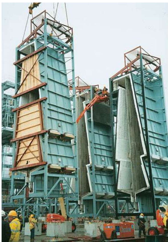
Figure 8.7 - Construction of a TWR
