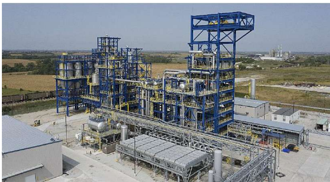
Figure 8.14 - Monolith Materials Emissions Free Hydrogen Plant, Olive Creek, Nebraska
