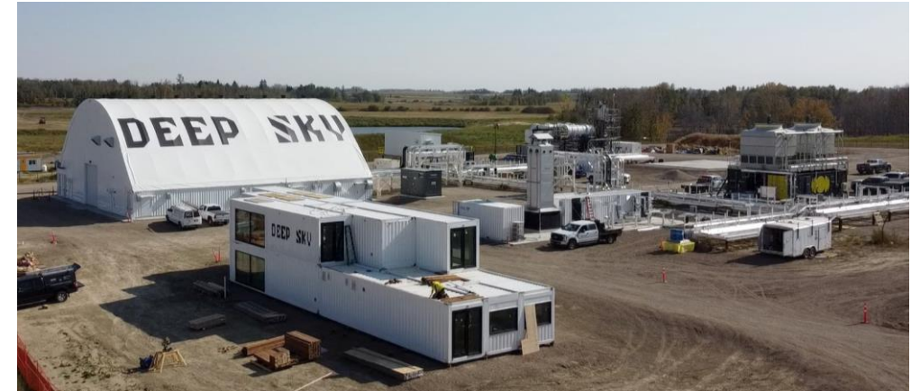
Fig 4.5-1, Deep Sky – Alpha facility. Source: Deep Sky
