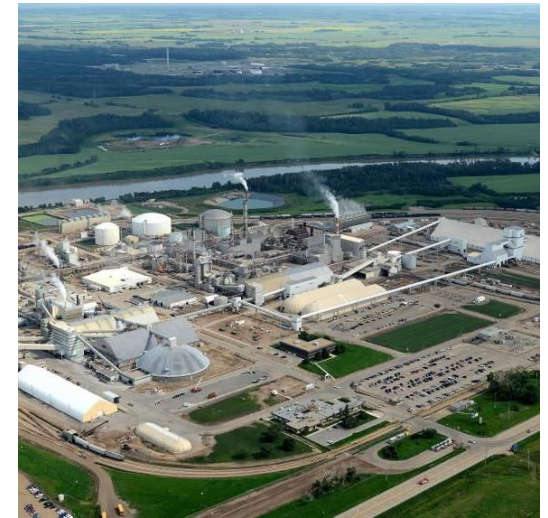
Redwater Fertilizer Facility, Alberta Canada
